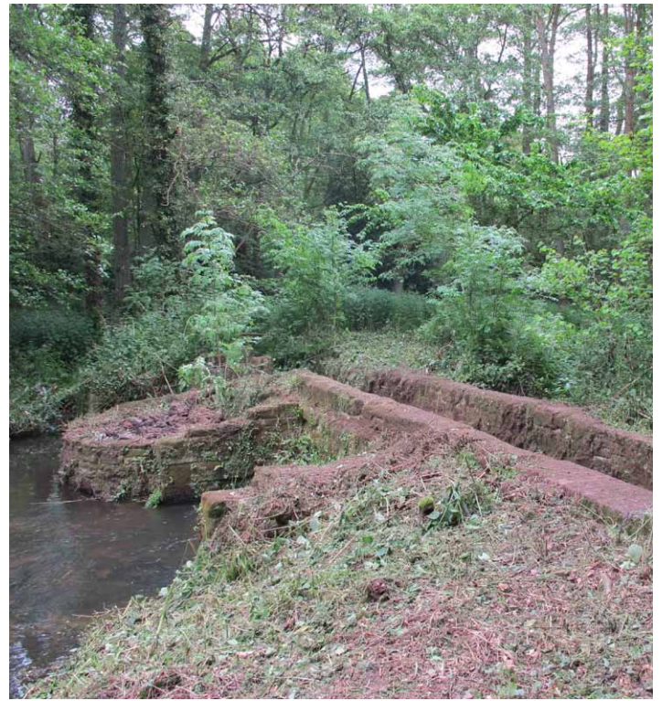
Fig 13. Aqueducts carried water through narrow sections of the Wey Valley, allowing its water meadow systems to function in difficult topography. This example at Bramshott Court is one of several built to connect water meadows on either side of the river.
