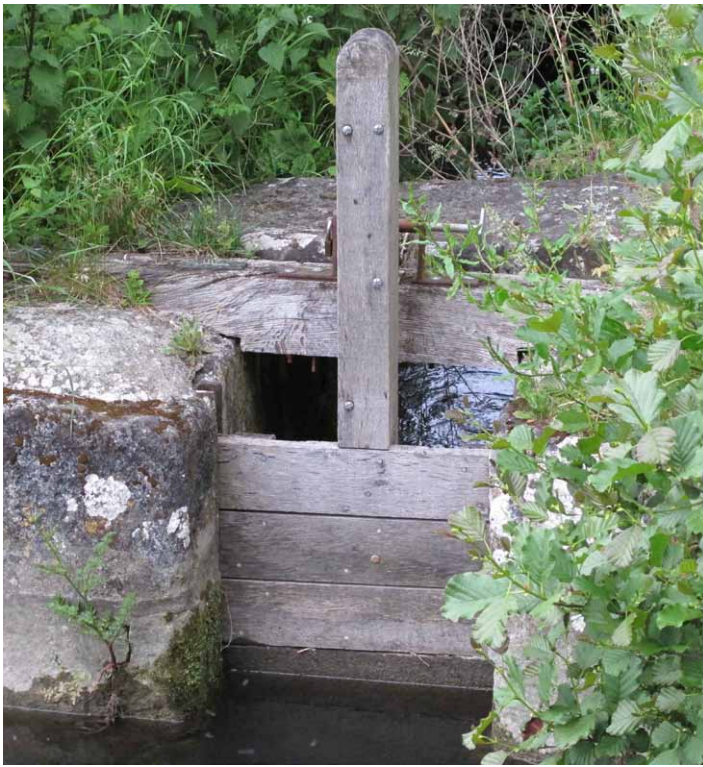
Fig 10. A restored water meadow hatch in use today at Harnham, Wiltshire.
